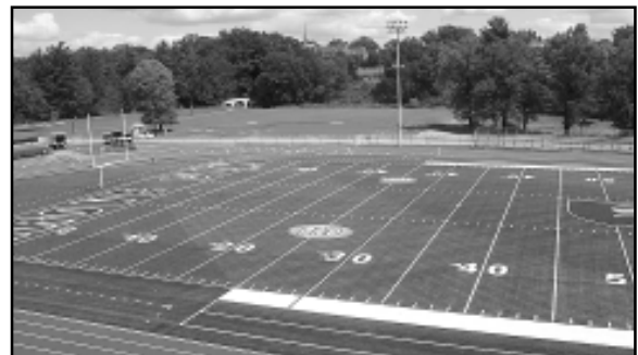
Grove City College installed lights, a new track and CSTurf at Robert E. Thorn Field during the summer of 2006.
